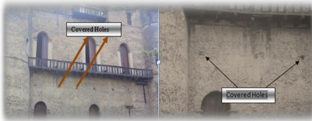
Figure 5: Covered holes for the wooden beams in the main Castel.
