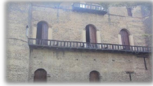
Figure 2: Buildings in good condition
