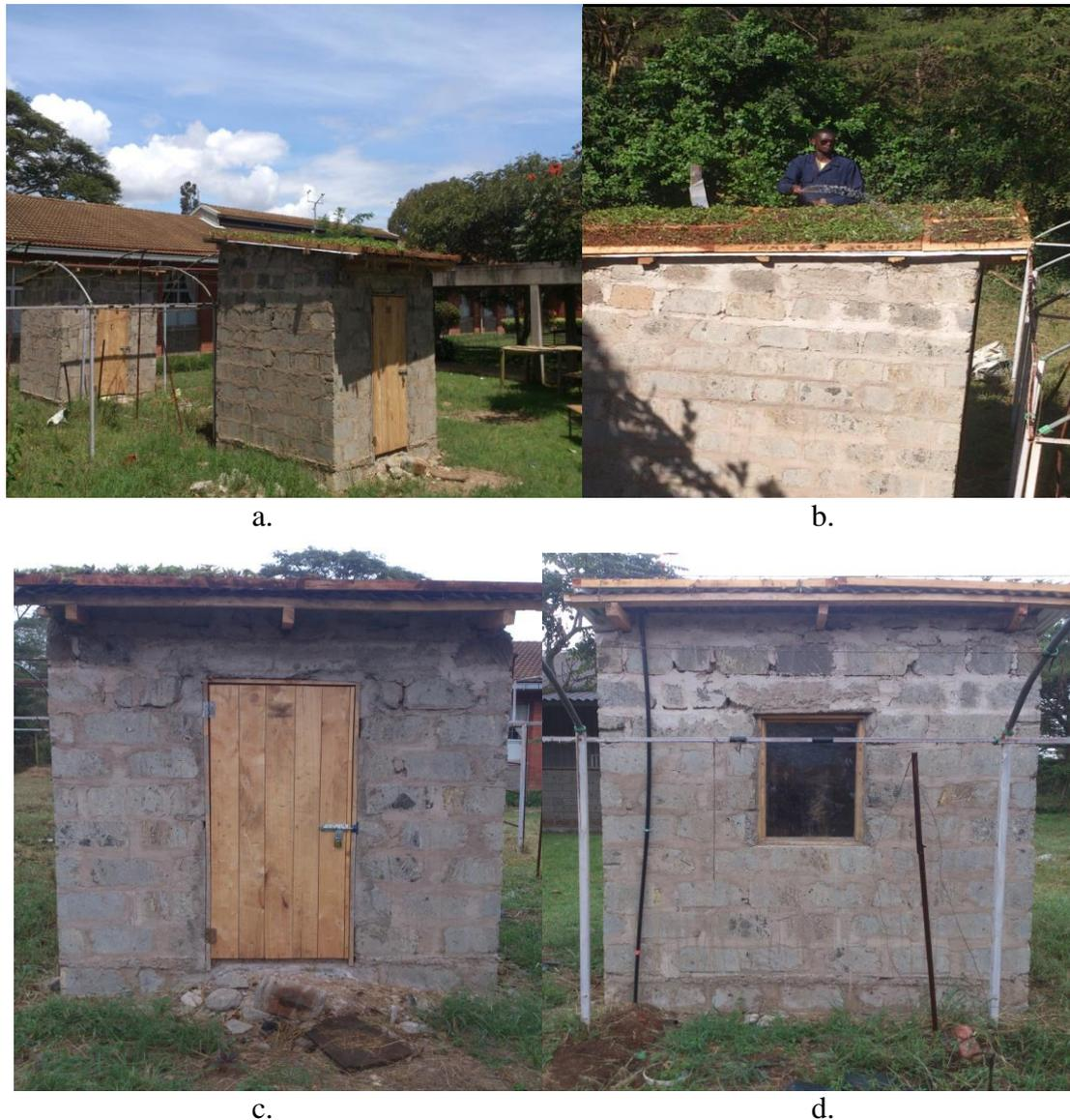
**Figure 1.** The different views of the field scale model (a) The full model. (b) The vegetation boxes on the roof. (c) The door. (d) The window (on opposite of the door).
