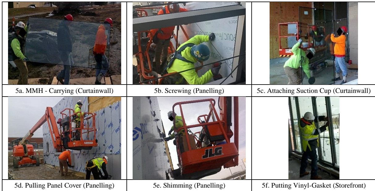
Figure 5. Glass/Panel installation
