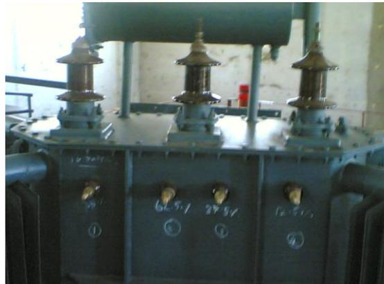
Figure 2 Transformer with tapped leads
