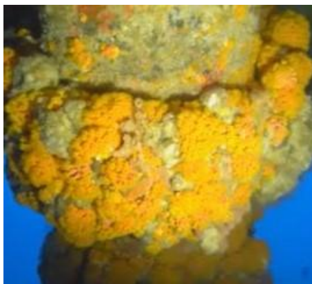
Figure 5: Elements of riser fouling from marine life. Adapted from [6].
