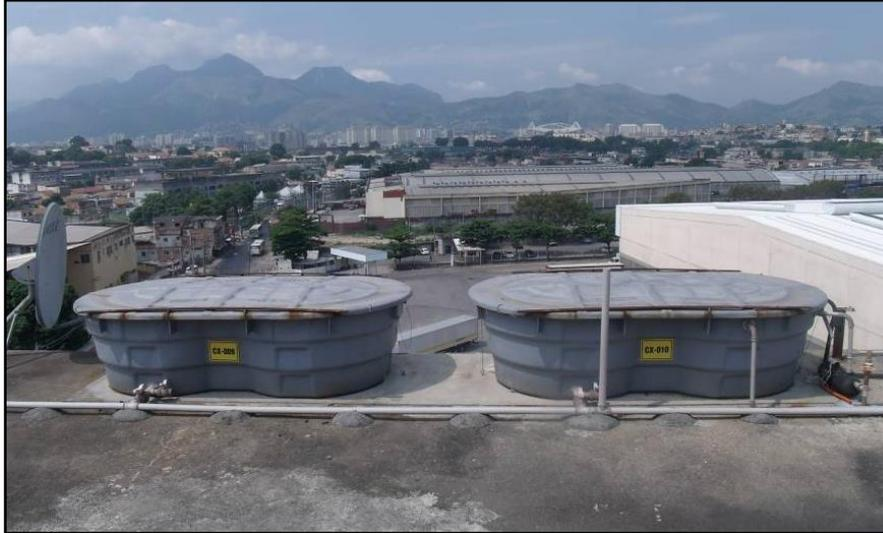
**Figure 8** - Water tank located on the roof of the factory continuously feeding the toilets.
