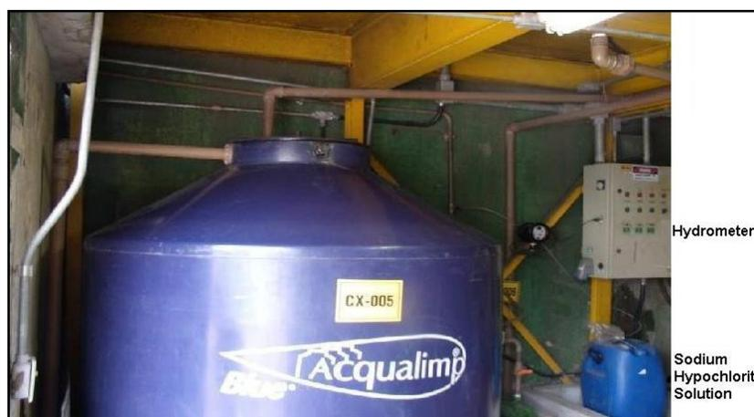
Figure 7 - Tank of 10,000 L and the treatment with sodium hypochlorite solution
