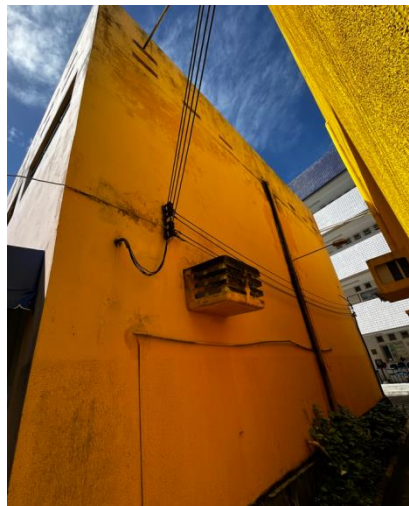
Figura 8. Right side facade of block G
