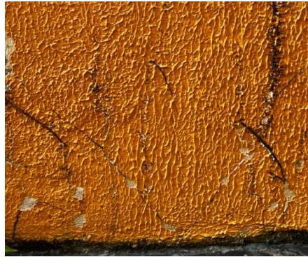
Figure 18. Paintwork detachment on the left lateral facade of block G
