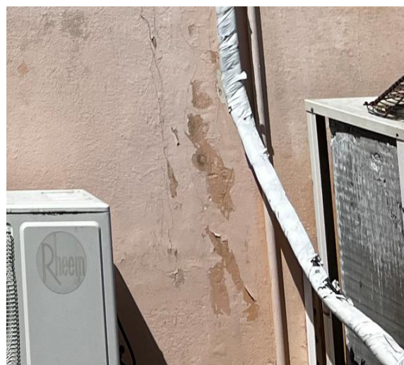
Figure 4. Paint detachment
