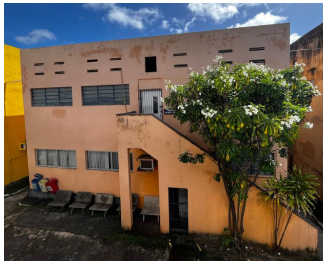
Figure 24. Rear facade of Block G
