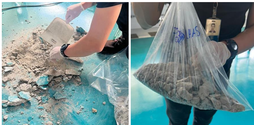
Figure 4 - On-site sample extraction procedure
