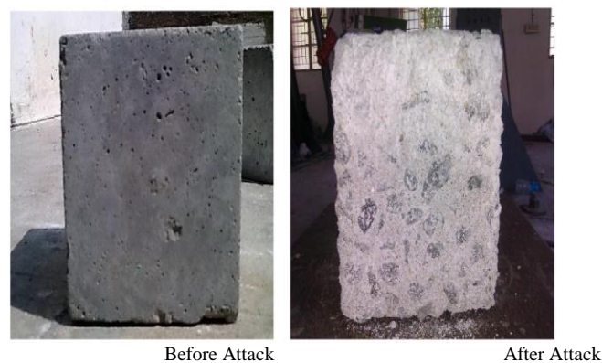
Fig.6. Result of Sulphate Attack
