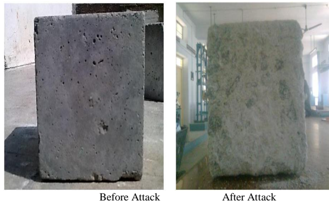
Fig.7. Result of Sulphate Attack
